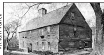
The 1677 Whipple house prior to 1927. This National Historic Landmark was restored and opened to the public in July 1899, as the earliest house museum in this country.
